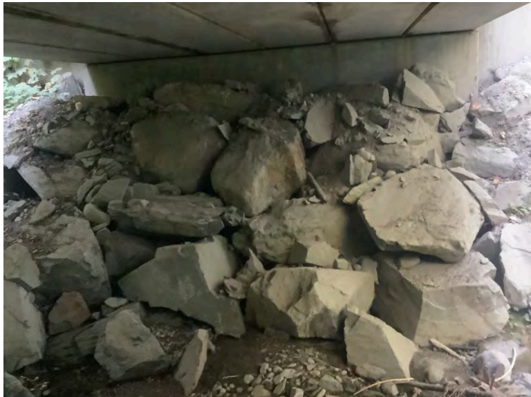
Left Bank Abutment when facing downstream
