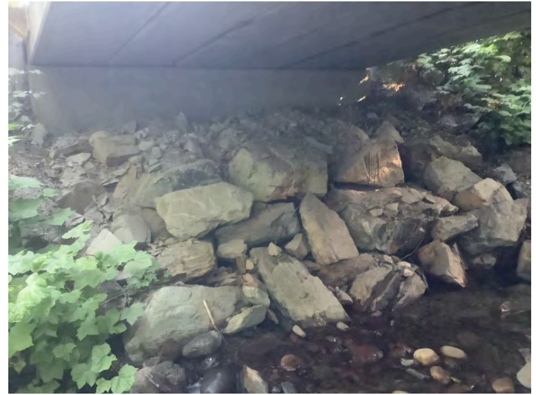
Right Bank Abutment when facing downstream
